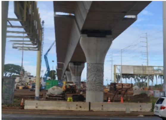
Sky Rail under construction in Hawaii
